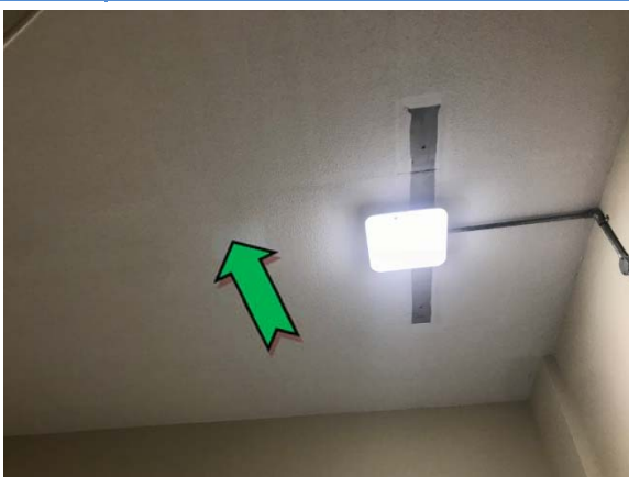
Photo 11. Interior, level 3, west elevation, staircase, ceiling – suspected non asbestos-containing textured coatings.
