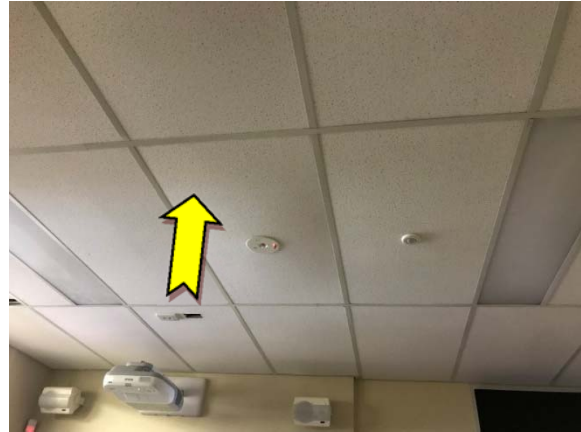
Photo 44. Interior, level 3, throughout, ceiling – suspected SMF compressed ceiling tiles.
