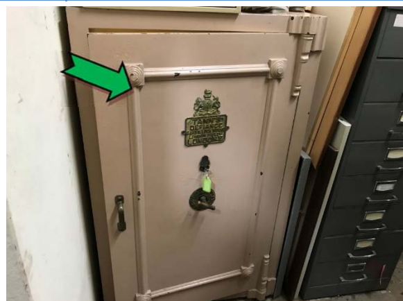
Photo 30. Interior, ground level, strong room, safe – suspected asbestos-containing internal insulation material.
