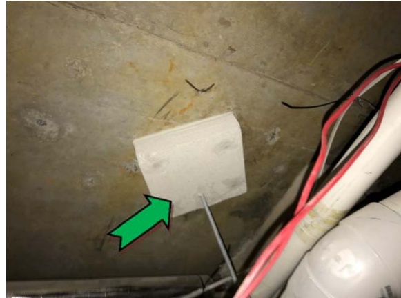
Photo 20. Interior, level 1, ceiling space – non asbestos-containing insulating board.
