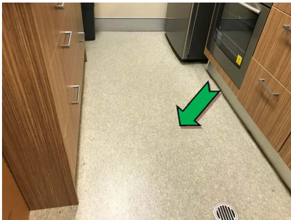
Photo 3. Interior, level 3, kitchen, floor coverings – suspected non asbestos-containing sheet vinyl.
