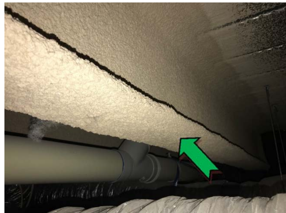
Photo 16. Interior, level 2, ceiling space, to support beams – non asbestos-containing insulation.
