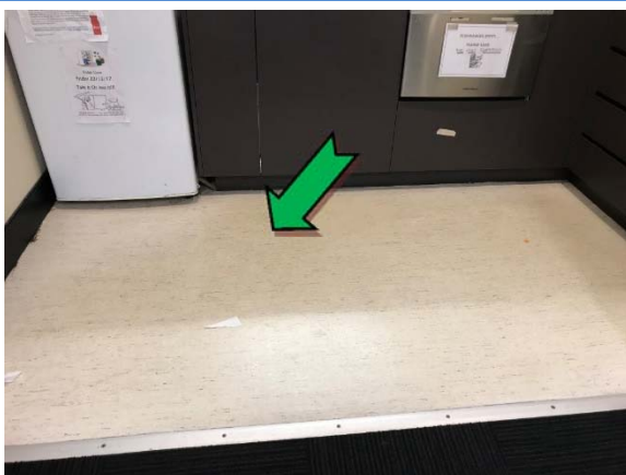
Photo 23. Interior, level 1, kitchen, floor coverings – non asbestos-containing sheet vinyl.
