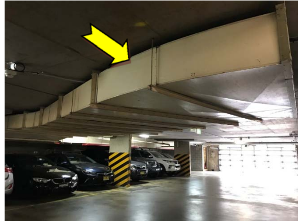
Photo 62. Interior, basement level, air condition ductwork – lead-containing cream upper paint system.
