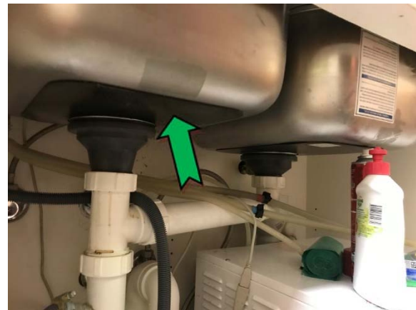
Photo 4. Interior, level 3, kitchen, under sink, sink pad – non asbestos-containing bituminous material.
