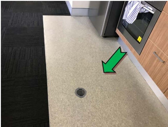
Photo 9. Interior, level 3, main office, kitchenette, floor coverings – suspected non asbestos-containing sheet vinyl.
