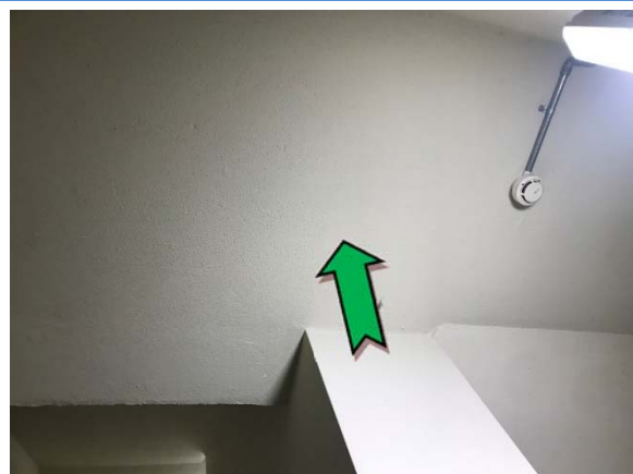
Photo 24. Interior, level 1, west elevation, staircase – suspected non asbestos-containing textured coatings.
