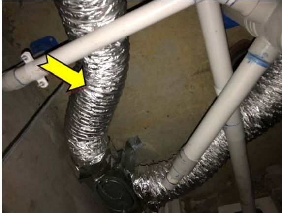
Photo 49. Interior, level 1, ceiling space, flexible ductwork – suspected SMF internal insulation.
