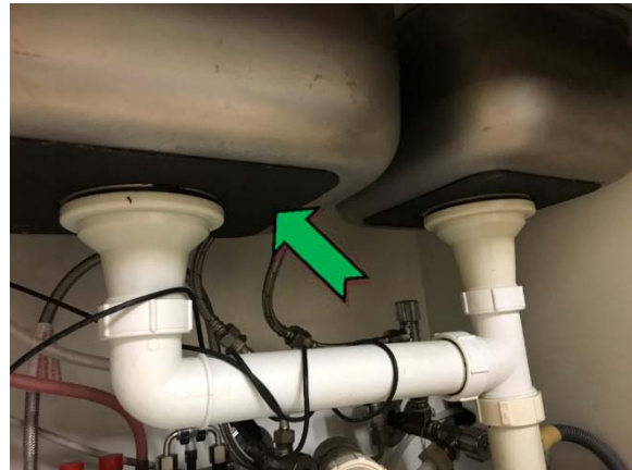
Photo 22. Interior, level 1, kitchen, under sink, sink pad – non asbestos-containing bituminous material.
