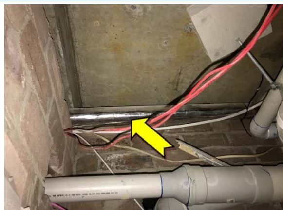
Photo 48. Interior, level 1, ceiling space, to pipework – suspected SMF external insulation.
