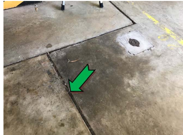
Photo 40. Interior, north-east corner, floor, expansion joint – non asbestos-containing construction joint mastic.
