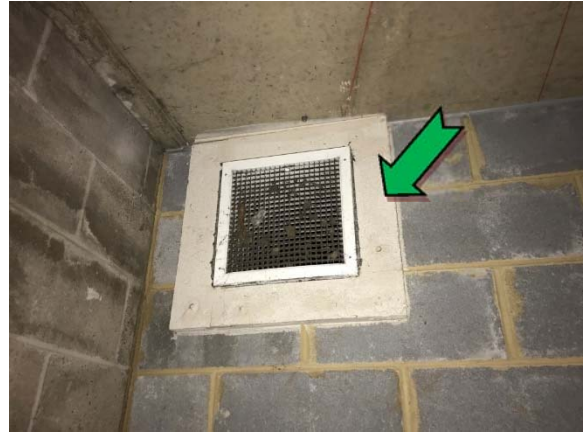
Photo 32. Interior, basement level, north-east corner – non asbestos-containing insulation board.
