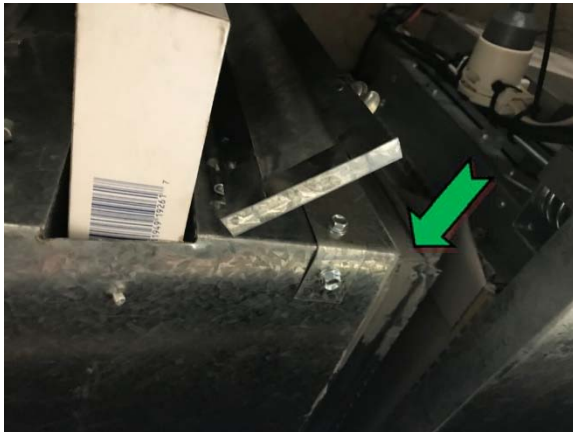
Photo 21. Interior, level 1, ceiling space, air conditioning ductwork – non asbestos-containing mastic sealant.
